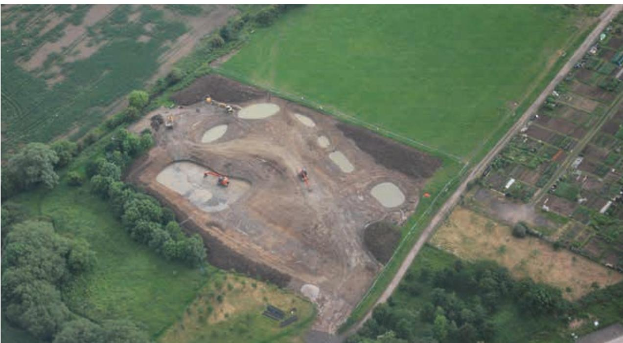
Fig 2. A large constructed wetland being constructed by Churchdown Council, Gloucestershire to enable untreated sewer water diversion and reduced local flooding. (Tamas Borandi, Water21)
